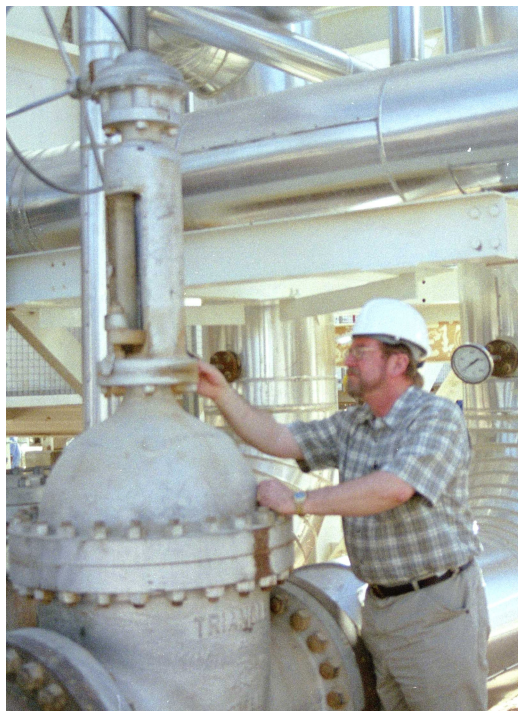
WILLIAM WHEATLEY ON SITE AT THE SAIH RAWL POWER PLANT
