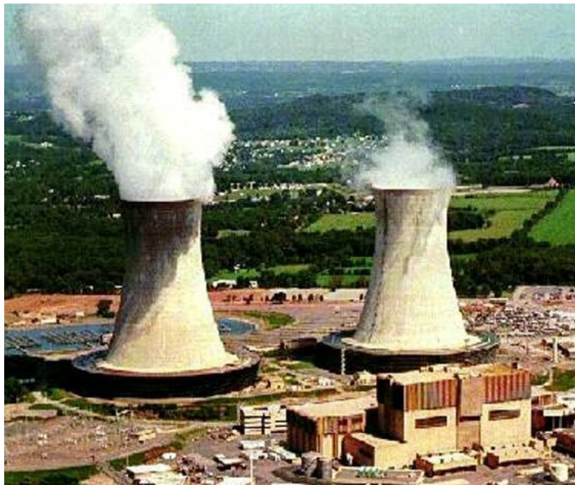
Limerick Generating Station
